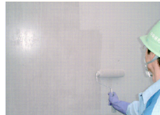
Taiheiyo ST-coating material containing photocatalytic \text{TiO}_2
